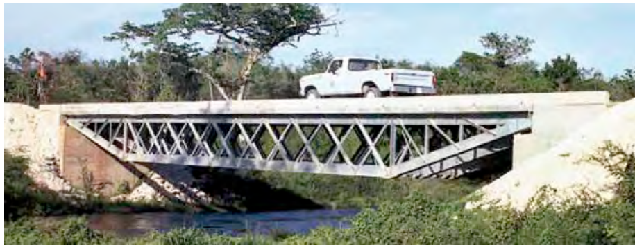
Steel frame truss bridge, located on the Southern Highway, Belize, Central America. Photograph © John Reid & Sons (Strucsteel) Ltd.
